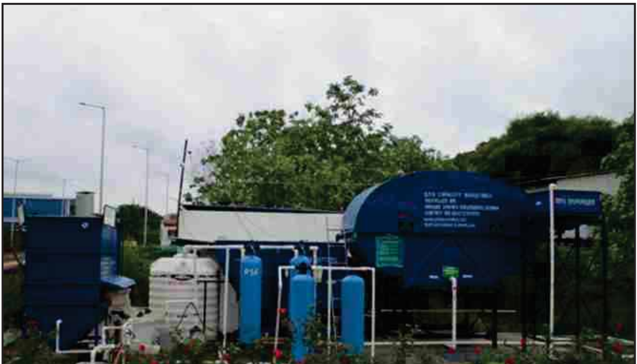
STP 50 KLD Capacity & ETP 2.5 KLD Capacity installed at Stamping Division to reuse waste water for plantation
